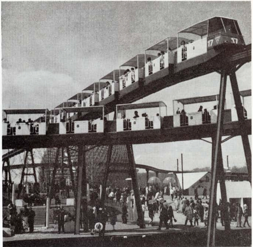
The power distribution contract for the Minirail system offered the greatest challenge. Britton Electric Ltd. did an excellent job.
